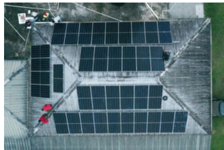
Below: New solar units now support operations at Alligator Head Foundation. © Giovanni Rimann, Rimann Renewables
